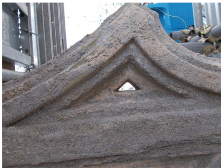
Figure 4. Candoglia marble stone unit damaged by weathering in AT6.
