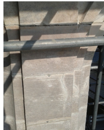
Figure 7. Vertical cracks on small pillars in AT8.
